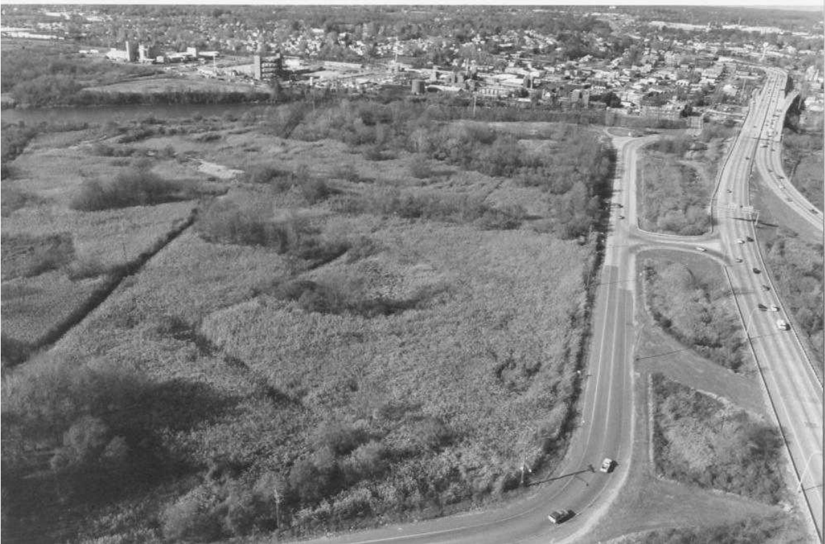
Figure 2-4 - South Wetland – Pre-remediation (looking from the S).
