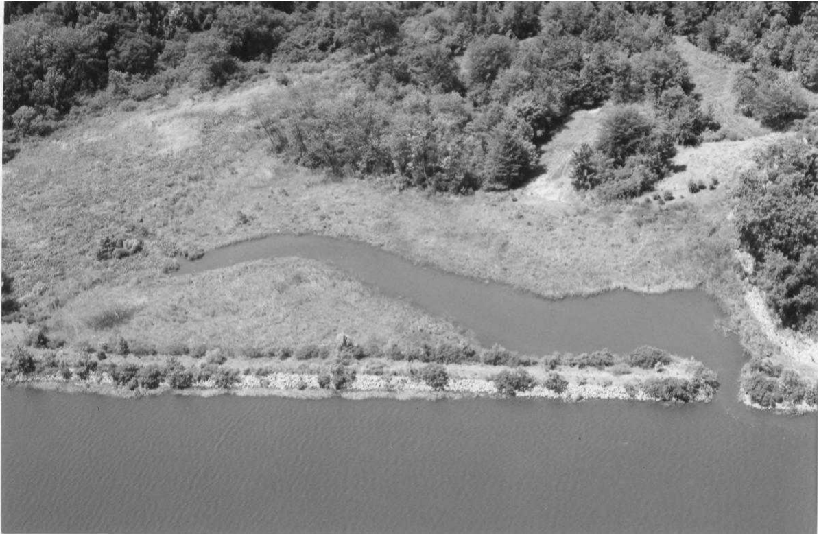
Figure 2-3 - North Wetlands – Post Restoration
