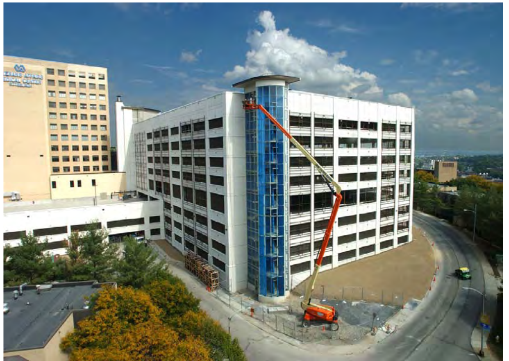
Exterior photo of the parking garage construction as it nears completion
