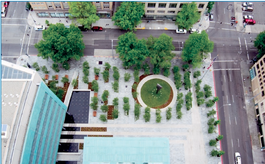
Figure 6-18: Overhead view of plaza, Seattle Court House.
