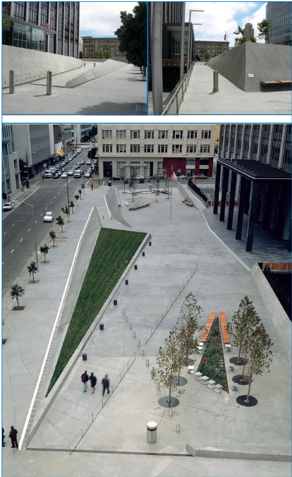
Figure 6-17: Sculptured forms, streetscape elements, and custom-designed bollards used as barriers at the San Francisco Federal Building.
