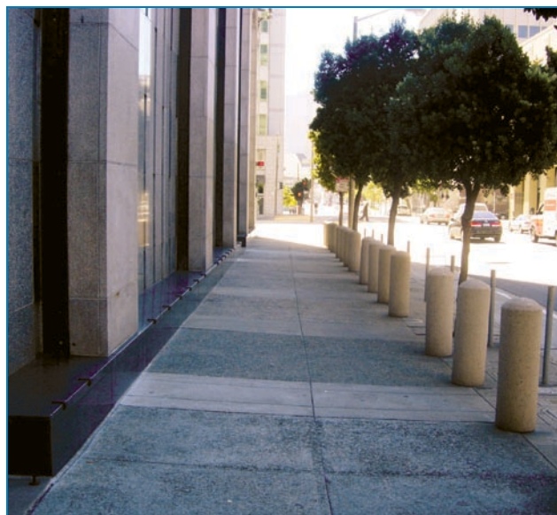
Figure 6-8: A well-designed zero-setback protection. The engineered bollards define the transition between the first and second layers of defense and the street trees soften the intrusion of bollards.
