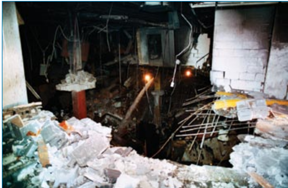
Figure 3-1: Damage in WTC garage caused by the 1993 bomb attack.
