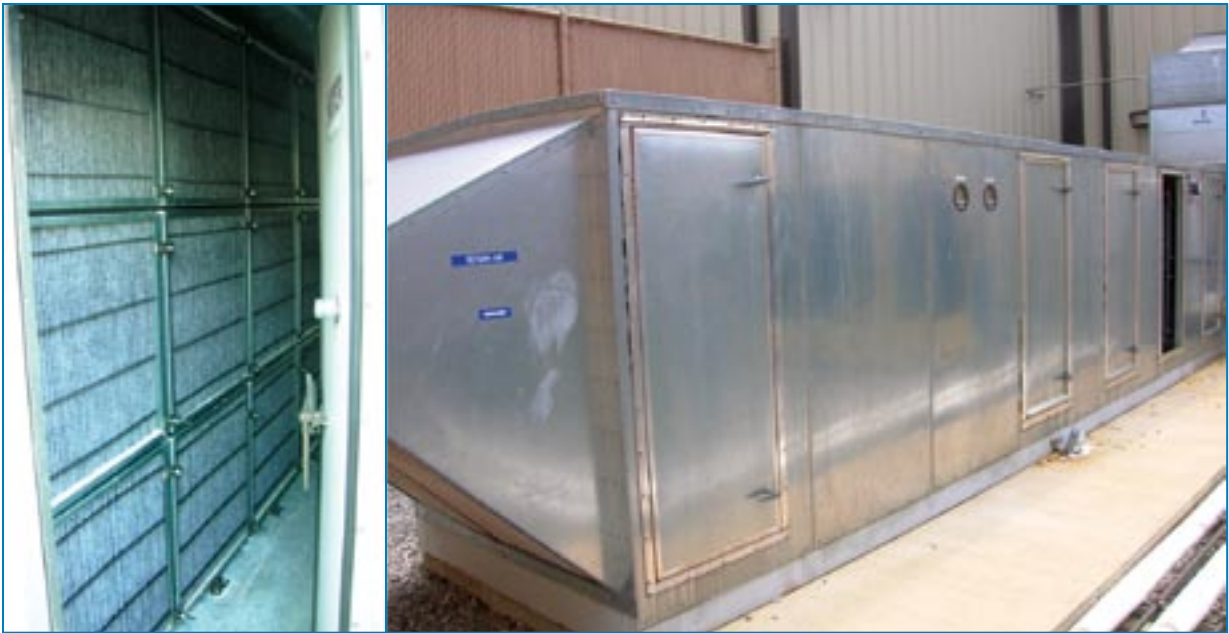
Figure 4-6: 9,000-cfm filter unit incorporating pleated adsorbers.
