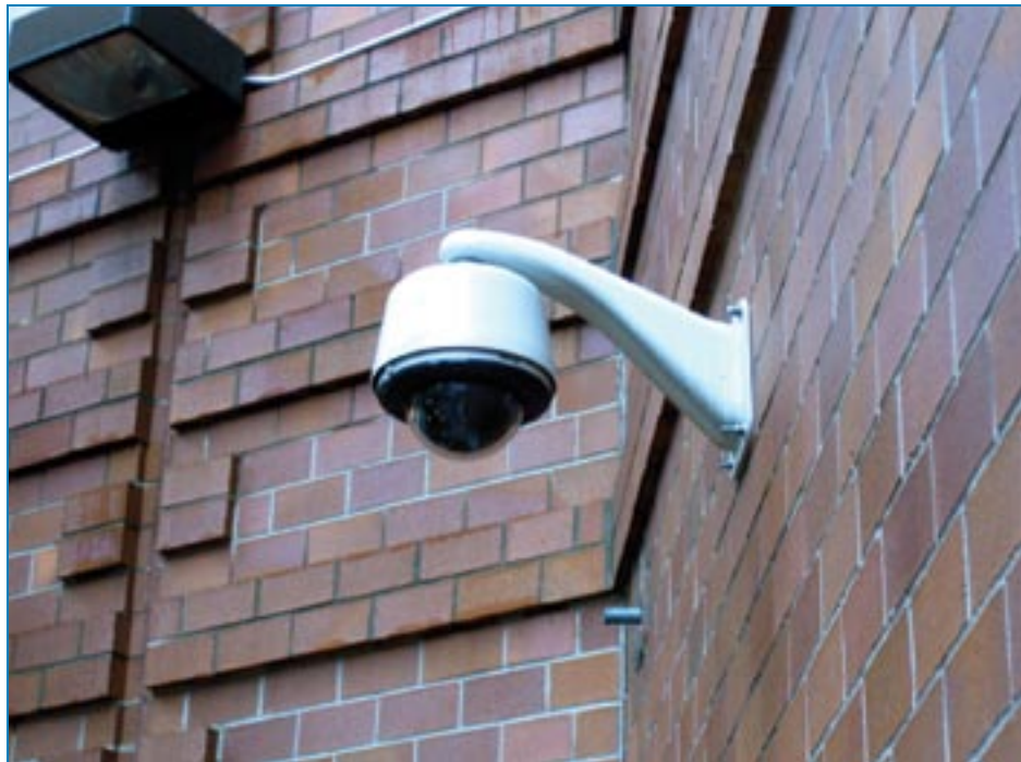
Figure 5-11: Exterior video camera for monitoring critical utilities.
