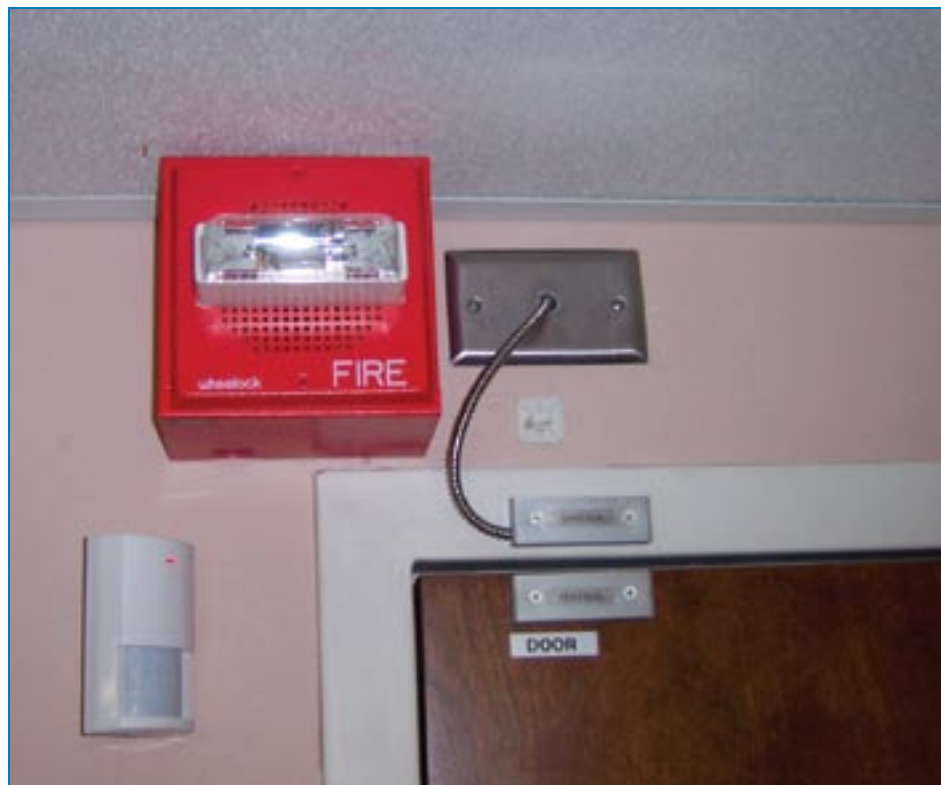
Figure 5-1: Doorway with balanced magnetic switch and passive infrared motion sensor.
