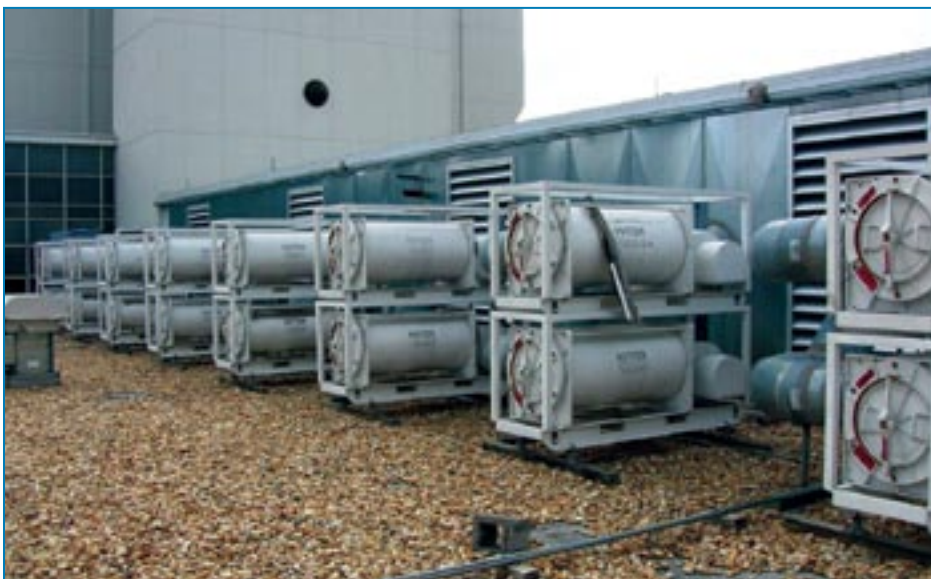
Figure 4-8: Radial-flow adsorbers in multiple 1,000-cfm housings in a 16,000-cfm system serving a hospital.
