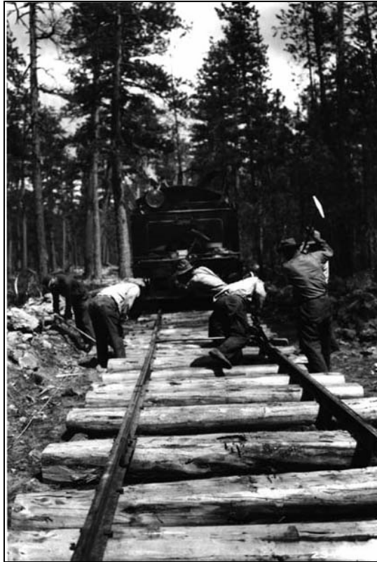
Figure 17: Laying Track for Shevlin-Hixon Logging Company
