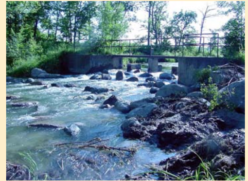
After Fish Passage Improvement
