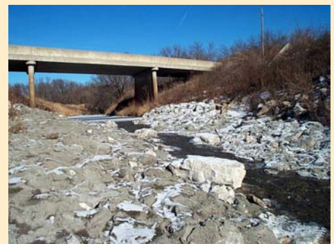
After Fish Passage Improvement
