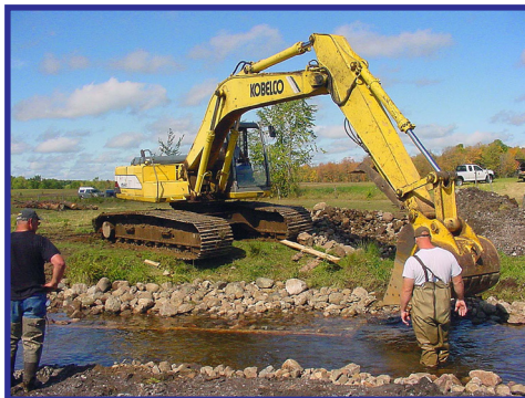
The Foytik stream restoration project eliminated cattle access to 1,500 feet of the Little Elk River. The river was returned to a natural meander with cattle access restricted to a rock crossing point (below).
