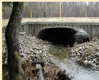
After Fish Passage Improvement
