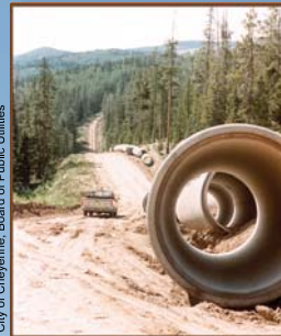
Six foot diameter pipe collects spring runoff on the west side of the Continental Divide.
