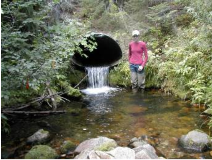
Figure 34 - Road 5662 culvert barrier on Coal Creek. August 2007
