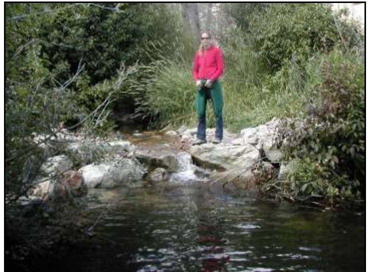
Figure 16 - Diversion for the Trollope-Hawkes irrigation ditch, after reconstruction. This is the uppermost of three boulder weirs.
