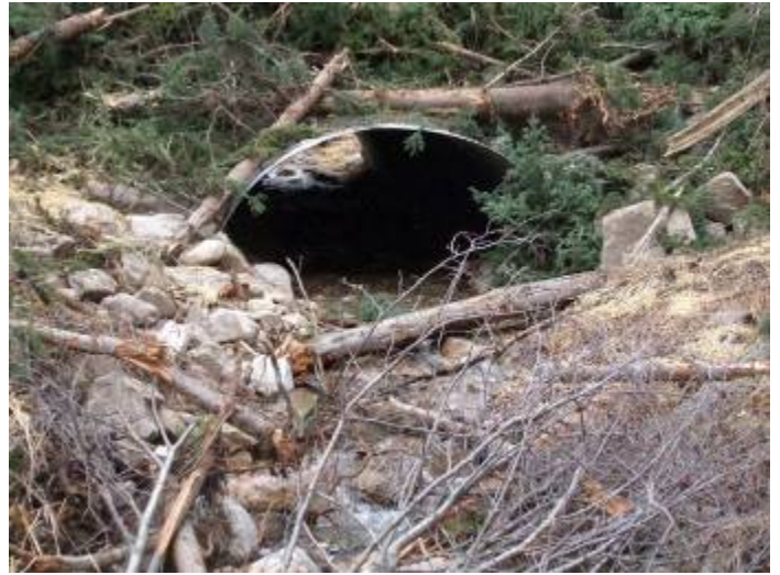
Figure 35 – Same crossing, after installation of a fish passable culvert. October 2007
