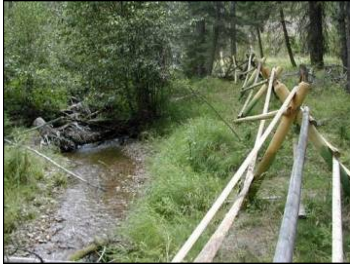
Figure 20 - Typical view of the Coal Creek jack-leg drift fence that was constructed in July 2007.
