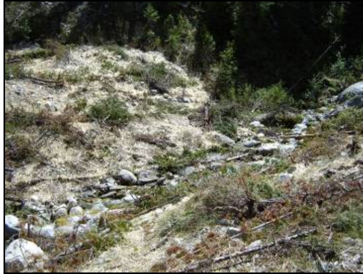
Figure 25 - Recontoured Road 74160 crossing of Coal Creek, 10 months after culvert removal
