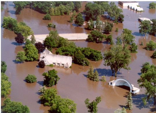
The flood-proofed, former St. Paul's Evangelical Lutheran Church withstood 2002 flooding. (Photo: Nate Howard, Post Bulletin)
