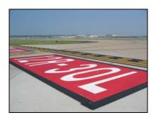
Surface Painted Holding Position Signs must be in accordance with AC 150/5340-1J, Change 2, Par 26.
