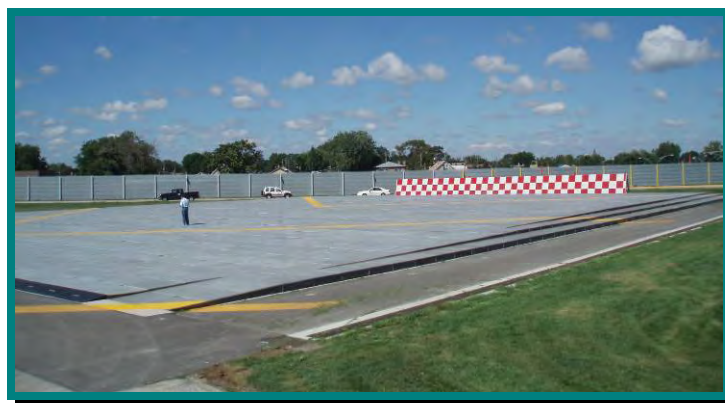
New EMAS installation at Chicago Midway International Airport.
