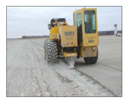
Figure 1. Resonant Breaker Machine
