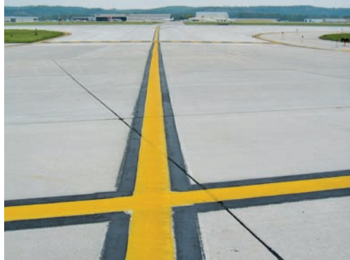
Figure 14 Enhanced Taxiway Centerline Markings
