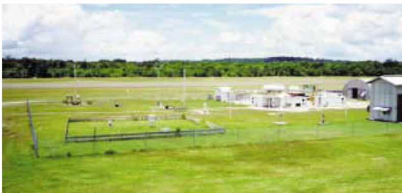
Figure 4. Manus Weather Station. The ARCS installation at the National Weather Service station at Momote airport, Manus Province, Papua, New Guinea.
