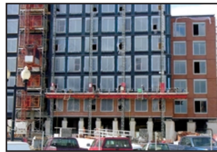
The Remsen Building, seen here under construction, is scheduled to be occupied in December 2003.
