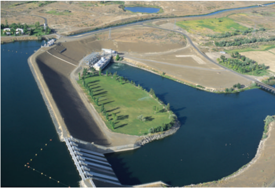
Left: C.J. Strike Dam, an earth dam of the hydraulic-fill type, is on the Snake River in Idaho and is 144 ft (44 m) high. David R. Frazier Photolibrary, Inc.
