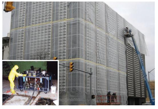
In a "dirty" bomb scenario, radioactive contamination may not be restricted to a building's exterior but penetrate deeply into its concrete. We are developing a model that predicts and optimizes how electrokinetics can be used to remove radionuclides from the concrete.
