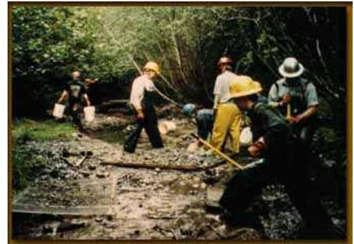
Sediment removal from channel
