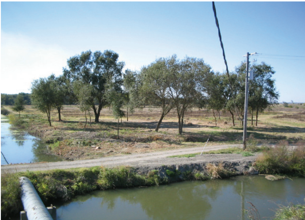
Tract 1, cell 1 west of lift pump after.
