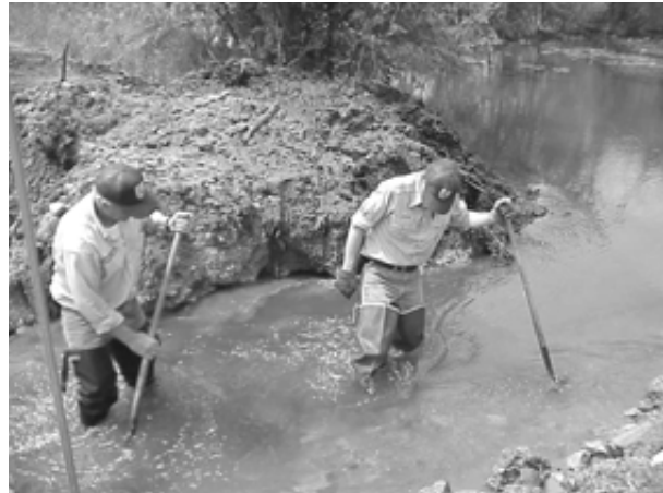
Culvert replacement at Trempealeau NWR. USFWS
