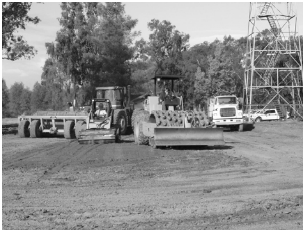
Construction of building pad at Sacramento Refuge Photo by Steve Emmons
