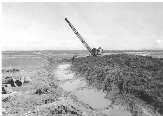
Constructing delivery ditches at Sacramento Refuge (1938) USFWS Photo
