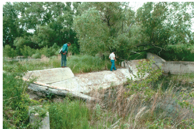
Service staff inspects a structure at Sheyenne Lake NWR.
