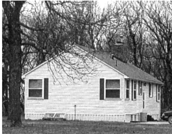
Refuge headquarters was constructed by a CCC crew in 1938-39. USFW
