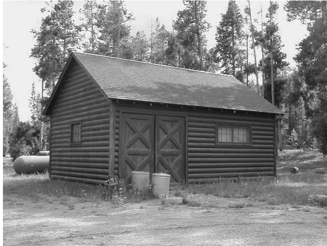
Photo: East Fork Blacks Fork Bunkhouse
