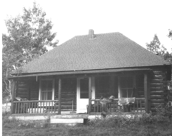
Hole in the Rock ranger dwelling, 1965.
