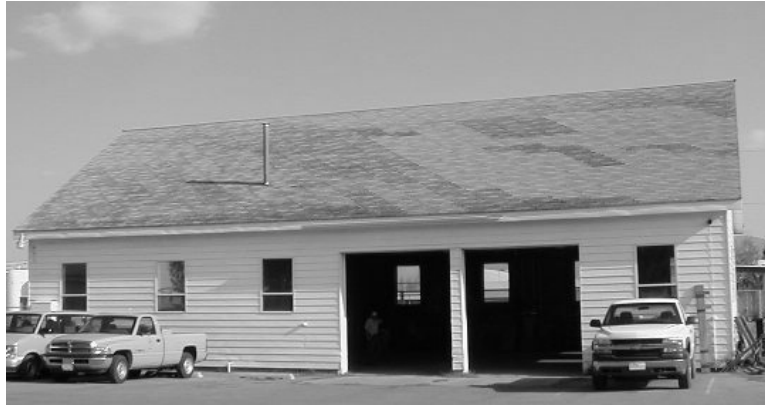
Photo: Kamas Warehouse
