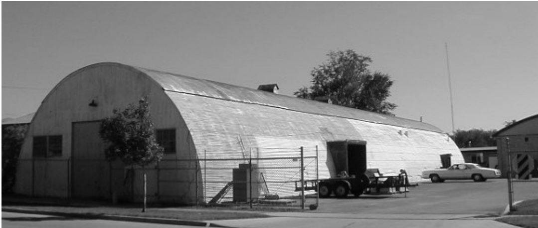
Photo: Redwood Warehouse
