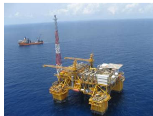
$ 2 Billion Oil Production Platform
