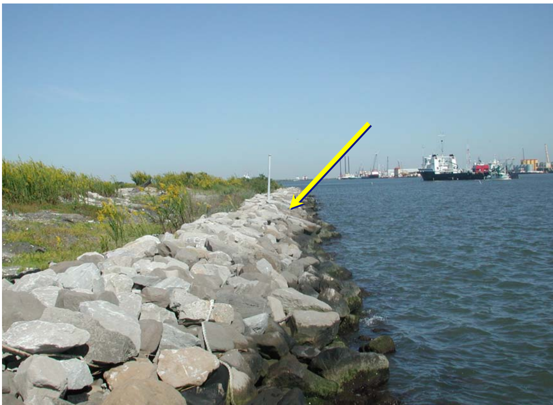
Figure 11-d. Ground photograph of riprap along Bayou Lafourche, a heavily trafficked waterway (October 2003). Note the steepness of the intertidal zone and the typical width of the structure.
