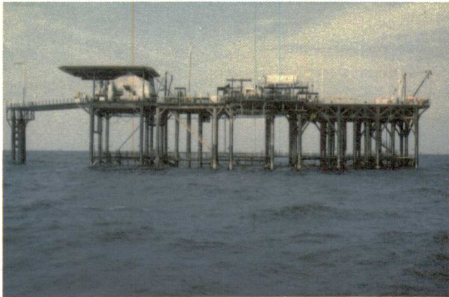
PLATFORM 2: BM3KN OPERATOR: Chevron LOCATION: 29^{\circ} 02' 50'' by 90^{\circ} 09' 46'' DATE INSTALLED: 1954
