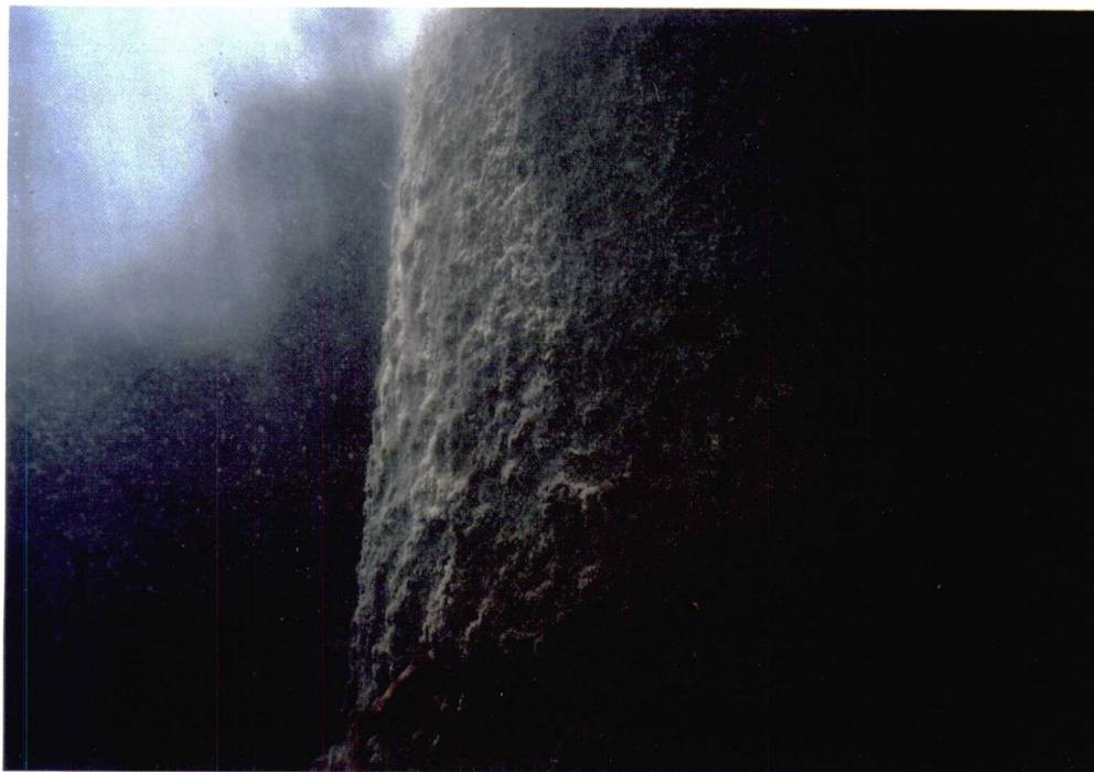
Affected area of biofouling community immediately below produced water discharge (seen in upper left). Photo taken at 1m water depth.
