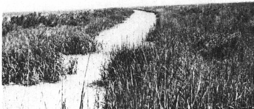
Figure 7.16. L24 line: push-pull ditch filled but unvegetated north of bulkhead. Spoil mounds are located to right and left of ditch.
