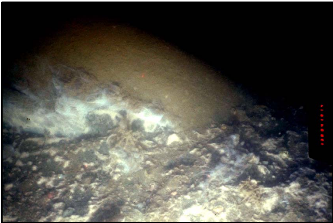
Photo 2-22 - Accumulation of suspected mud and cuttings near the base of a Main Pass 288 platform diagonal support. White filamentous mat (? Beggiatoa spp.) is conspicuously visible adjacent to the platform support structure.
