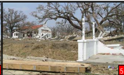
Damage and debris from Hurricane Katrina at the VA Medical Center in Gulfport, MS illustrate another case for when IT and telehealth can provide support for 'brick and mortar' facilities (photos 4., 5. courtesy of Cary Parks IRM Chief, Hampton, VA)
