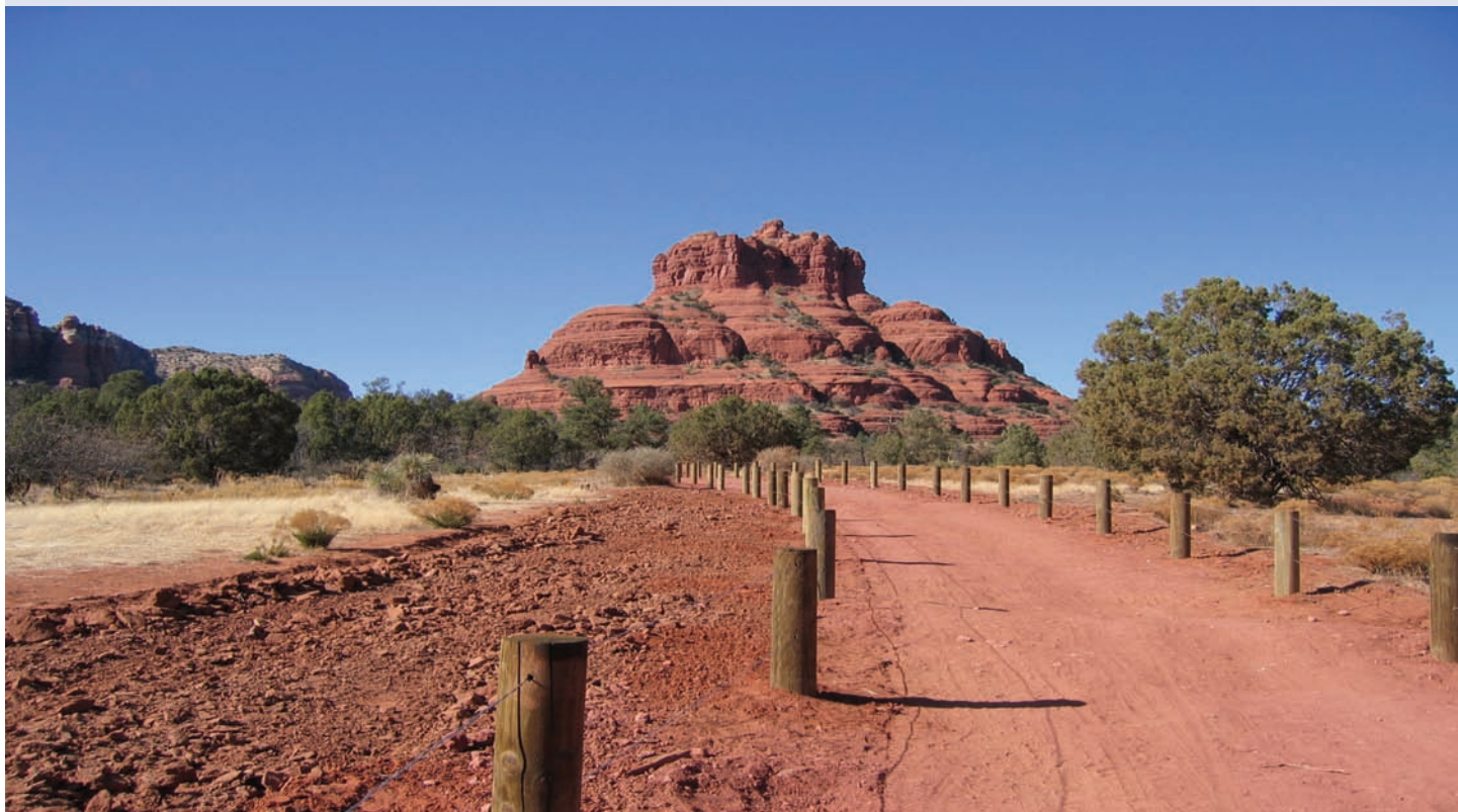
Bell Rock Pathway rehabilitation project
