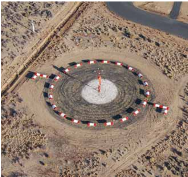
Figure 10-5. Left hand pattern for one direction and right hand pattern for other direction.
