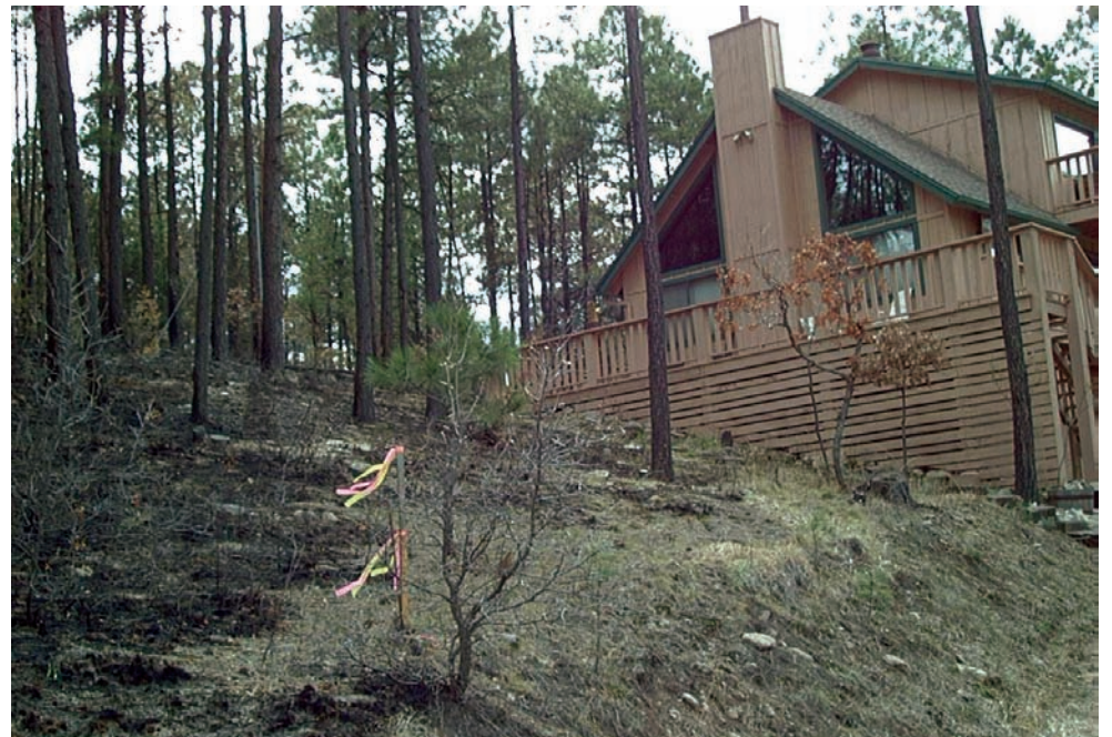
The pre-fire activities implemented by this homeowner include a maintained landscape, use of Firewise plant materials, reduced vegetation around the perimeter of the property and fire-resistant roofing material.
