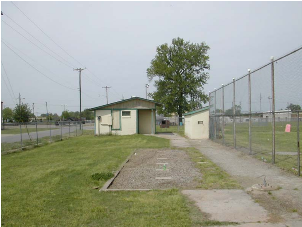
Photo 22 - Looking west at restrooms, dugout and landscaping in the southern portion of the site. South D Street is visible to the south.
