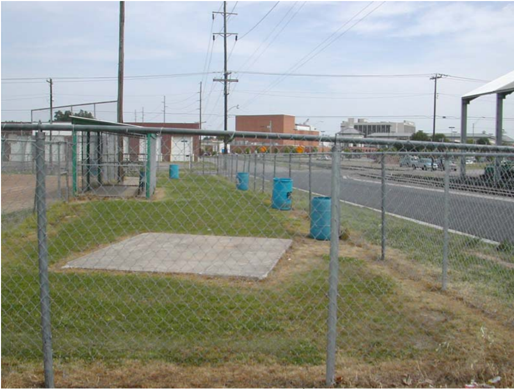
Photo 19 - Looking north at concrete pad along South 7 th Street.
