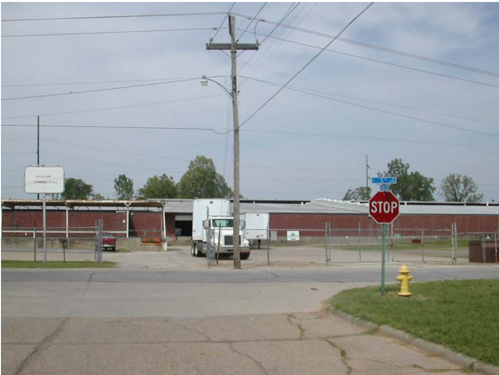
Photo 4 – Looking west at adjacent structure from the corner of South 5 th and South B Streets.
