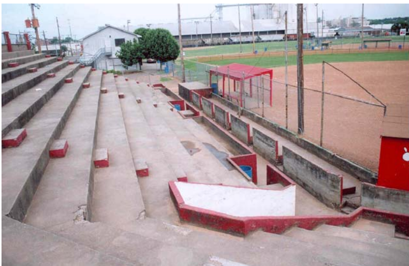
Photo 5 - Detail of Bleachers, Facing East
