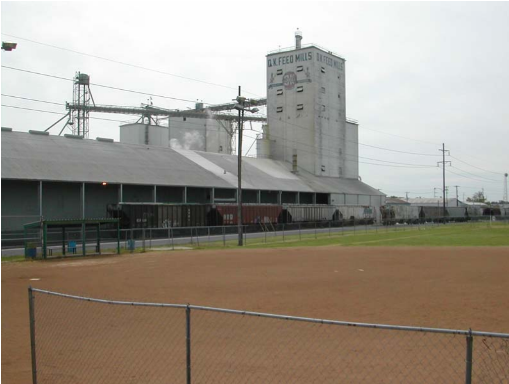
Photo 17 - Looking southeast at adjacent industrial structure (O.K. Feed Mills) and railroad.
