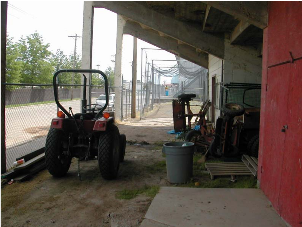
Photo 30 – Maintenance/storage area beneath Andrews Field grand stands. Materials and equipment for maintenance of the fields are stored here.
