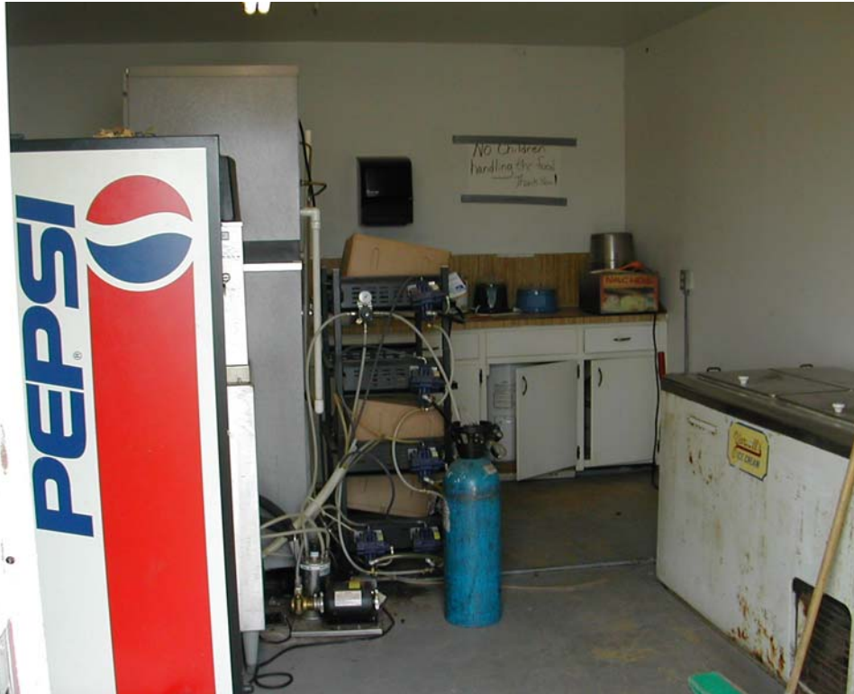
Photo 7 – Interior of a concessions building located in the southwest corner of the Andrews Field complex.
