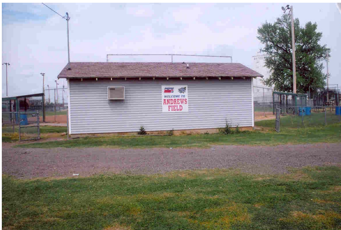
Photo 6 - Late 20 th Century Structure at the Southwest Corner of 9-Acre Tract, Facing Northeast
