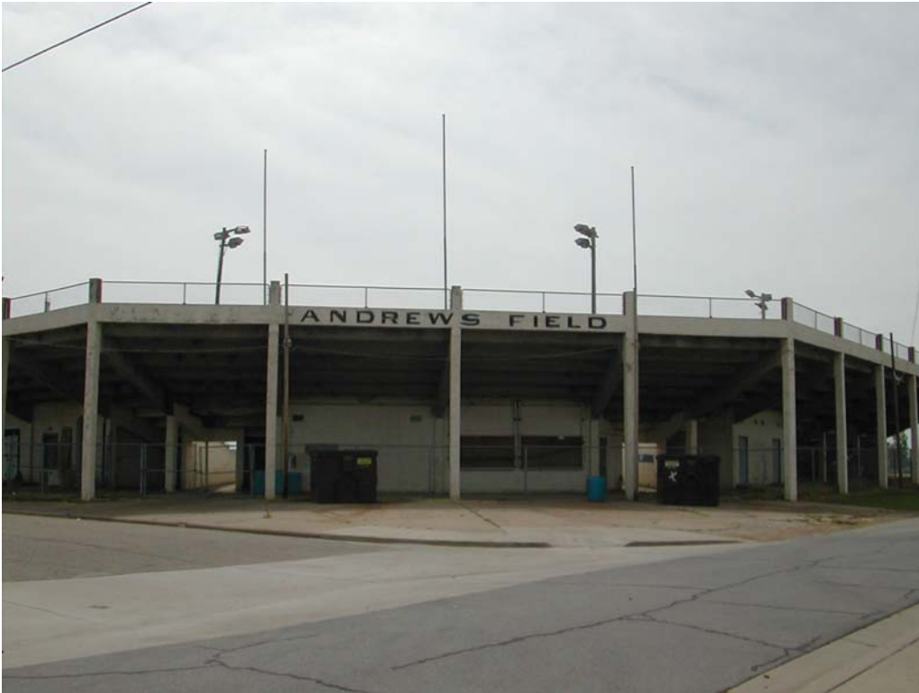
Photo 1: Looking southeast at the Andrews Field grand stands from the corner of South 5 th and South B Streets.
