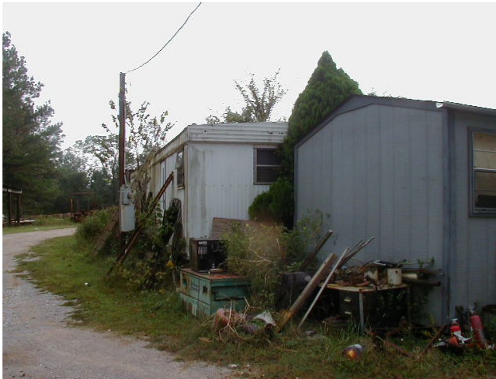
Photograph 5: View of house structures on the Jackson Tract, portion of Alternative A. September 29, 2005.
