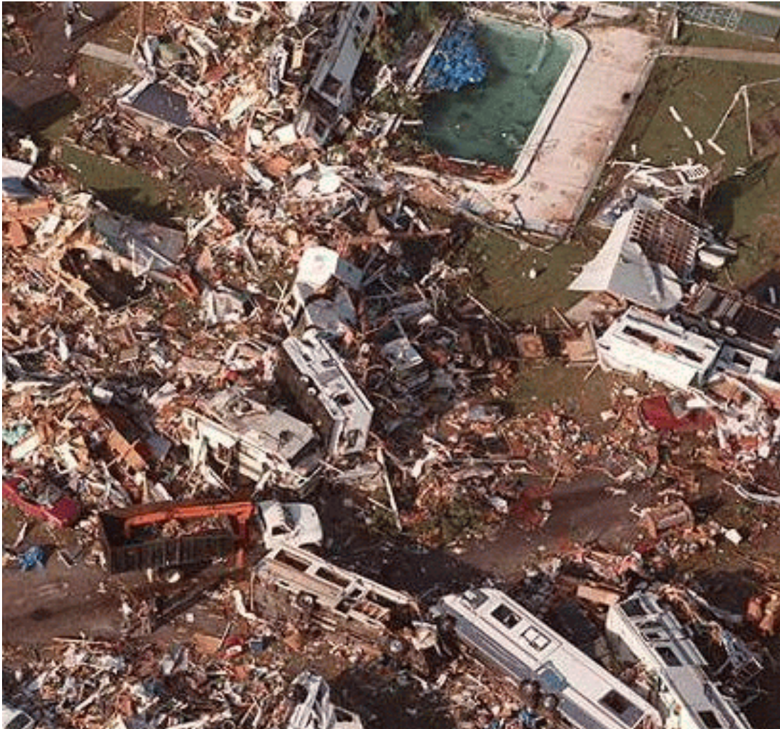
Aerial view of tornado damage to an RV park in Kissimee, Florida in February, 1998.
