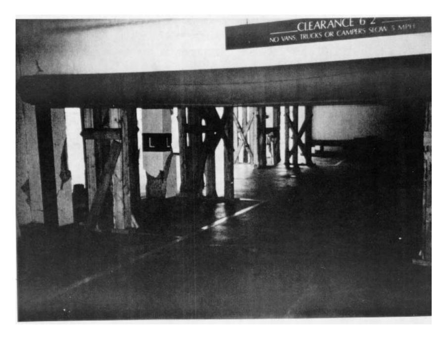
Example of shoring techniques used by the LAFD and the LACFD to prevent a secondary collapse of the high-rise hotel parking garage.
