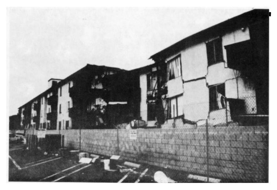
Collapsed portion of Northridge Meadows Apartments. Due to the soft story construction, the structure not only collapsed, but shifted 10 feet.
