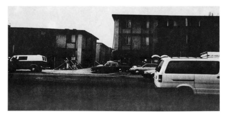
Initially firefighters thought that the Northridge Meadows Apartment building was a two-story structure. The building on the right is the original height of all the apartments.
