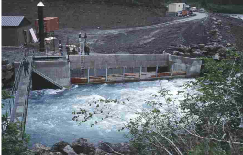
Figure 2.18: Power Creek diversion dam and intake.
