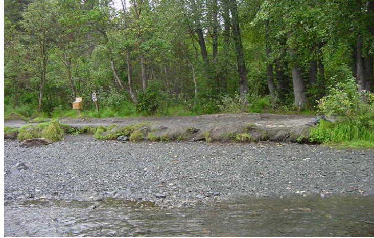
Figure 4.8: Trampled, compacted, and eroding streambank near the mouth of the Russian River (photo by Dean Davidson, Chugach National Forest).
