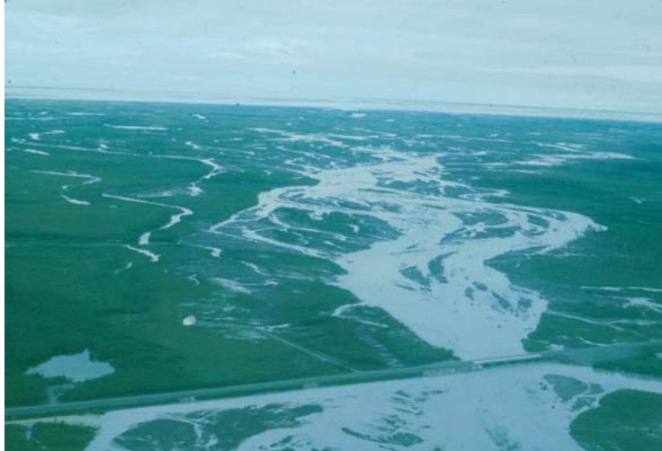
Figure 2.14-Copper River Highway bridge over the Sheridan River, view downstream. The bridge restricts channel migration downstream of the highway (August 1982).
