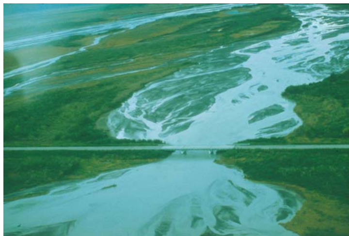
Figure 2.12-Copper River Highway Mile-8 Bridge over a channel of the Scott River, looking upstream. The bridge constricts the flow considerably (September, 1984).
