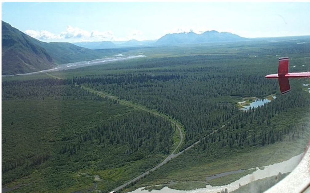
Figure 2.29 – Constructed portion of Carbon Mountain Road, across Clear Creek to Sheep Creek drainage. Photo taken August 2003.
