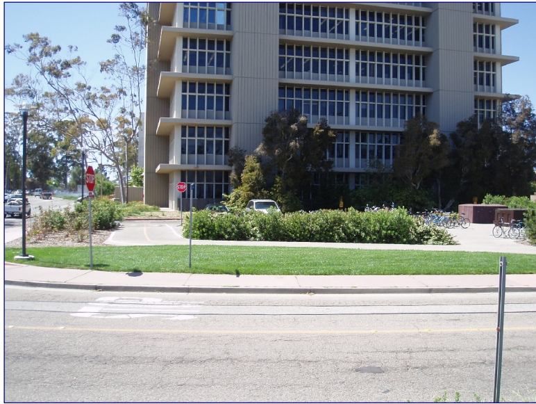
6(c) Southern Portion of Site (Looking West)
