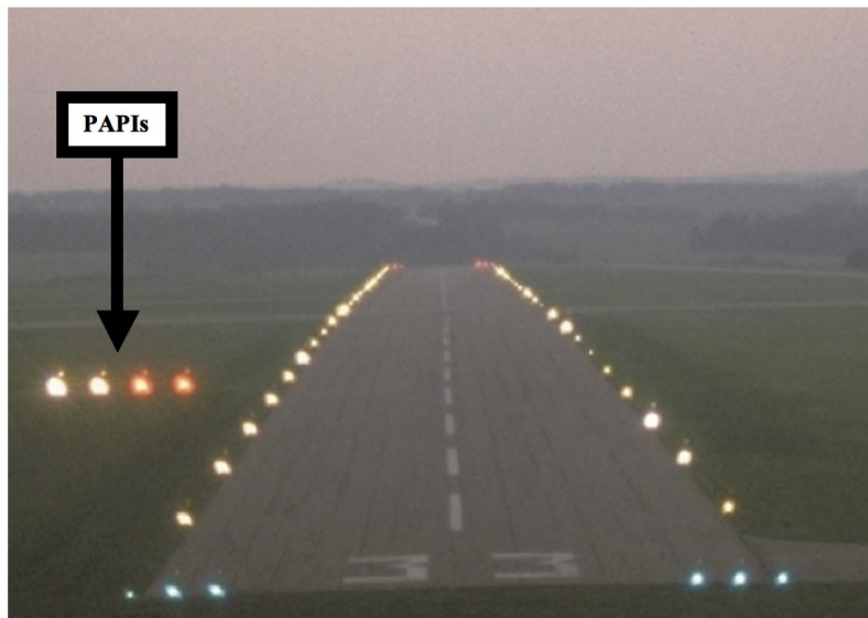
Figure 3. PAPI Light Fixture showing glide path information
