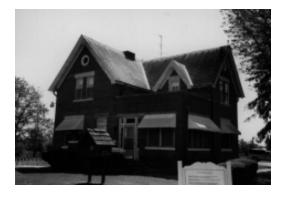
The lodge has a gable roof rather than the mansard typical of the Meigs lodges built in the 1860's and 1870's. The roof is slate. The windows, typical of the period but unusual in Meigs buildings, are double-hung with the lower panel having two panes with one vertical mullion and an upper panel with one central pane surrounded by 12 six-inch square panes.
