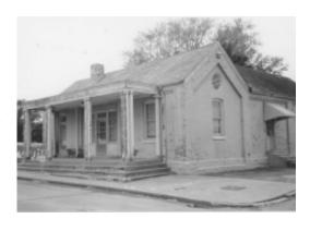
Adjacent to the former administration building is a brick and concrete tool house and garage, constructed in 1872. The roof is asphalt. In 1935 a brick and concrete addition of 33 feet by 22 feet, which included a basement, was constructed. The roof of the garage was replaced in 1963 with asphalt felt and self-sealing composition shingles. Three overhead metal garage doors were installed in 1965. This building is now used for storage.
