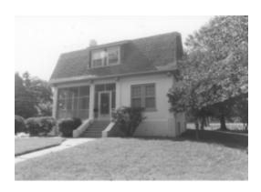
In 1928, the lodge was constructed. It is a one-and-one-half-story, six-room, brick and stucco building with a gambrel roof. The roof is fiberglass shingles. The lodge is located within the area of the semicircular projection on the east side of the cemetery.
