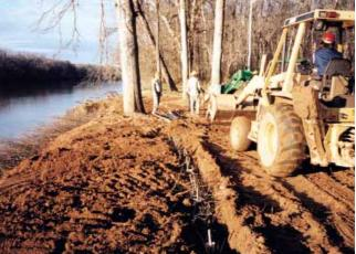
Another cribwall/brush layer was finished with a live fascine at the top of the bank. Note the brush layers extending toward the water.
