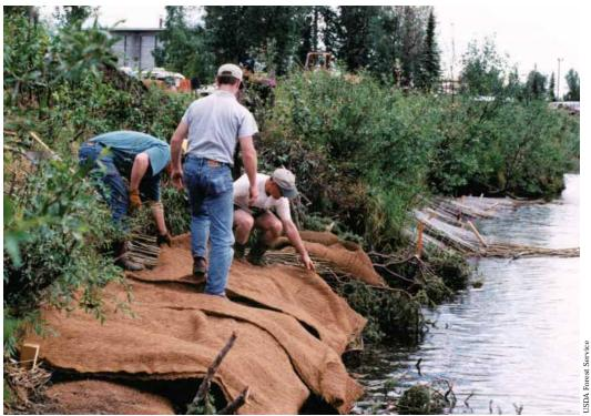
Vegetated geogrid—Coconut mat is laid over the tree revetment and rock. One foot of soil will be shoveled on top of the mat to begin a vegetated geogrid.
