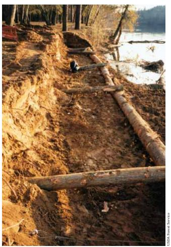
The first log of a cribwall is laid and anchored into the bank with a deadman.
