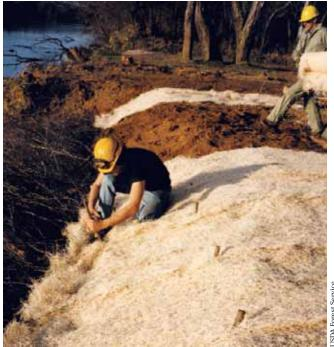
One cribwall/brush layer was finished using erosion control fabric and seeding.
