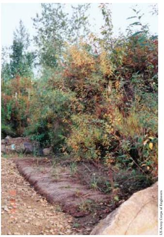
The lift was plugged with transplanted sedges from the riverbank. The sedges and the mat are trapping sediment and rebuilding the bank.
