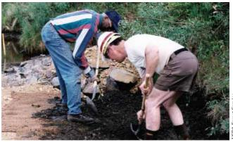
The beginnings of a plant lift. Soil was shoveled on top of a portion of the erosion control fabric. The loose end was folded over the fabric and staked, creating a lift.
