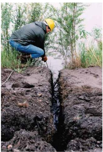
Cable leading to the tree revetment in this ditch is anchored to a metal pipe used as a deadman. The pipe is in a ditch perpendicular (in the foreground) to the one leading to the river.
