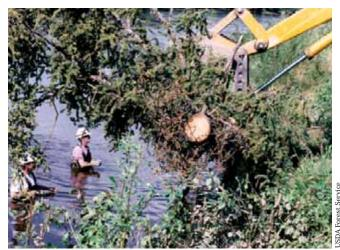
Excavator lowering a tree log into the river to be used as part of a tree revetment.
