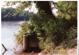
Downstream end of one cribwall keyed into a large tree.
