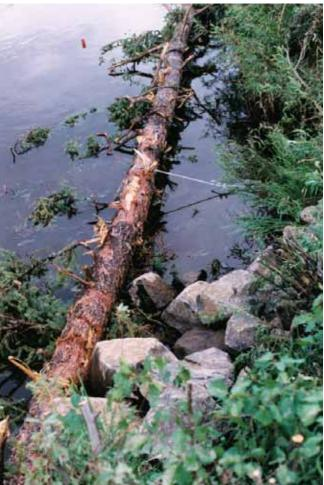
Two trees were stacked to form this revetment. The space between the bank and the trees was filled with rock.
