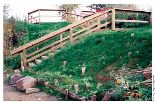
Stairs were built leading to a rock fishing platform. Three lines of fascines, erosion control fabric, and seeding stabilize this recontoured bank.
