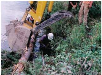
Excavator holding the tree log in place while it is attached by cable to the deadman in the bank.
