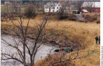
This 90-degree bend was stabilized using log revetments, root wads, live fascines, and live posts. It has withstood a 100-year flood event and ice flows. The visible flat area, formerly a cornfield, has been planted with riparian tree species. Two-foot squares of plastic were placed around the bases of the plants to control weed growth. Mad River, VT.
